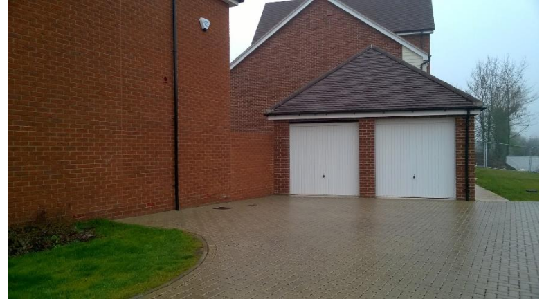
Permeable paving, Aylesbury
